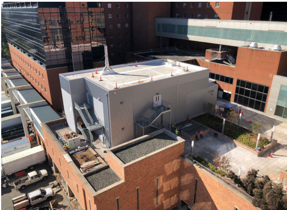
The Modular Terrace Facility will be used to produce cutting-edge cell and gene therapies for clinical research trial patients.
