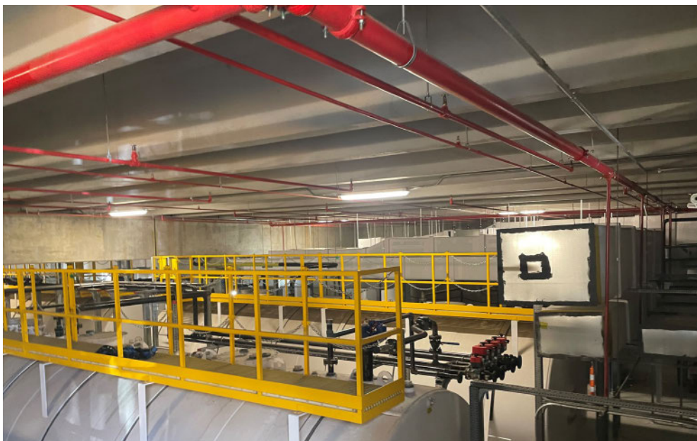
The ESSEG's generators can support the NIH Clinical Center for at least four days.
