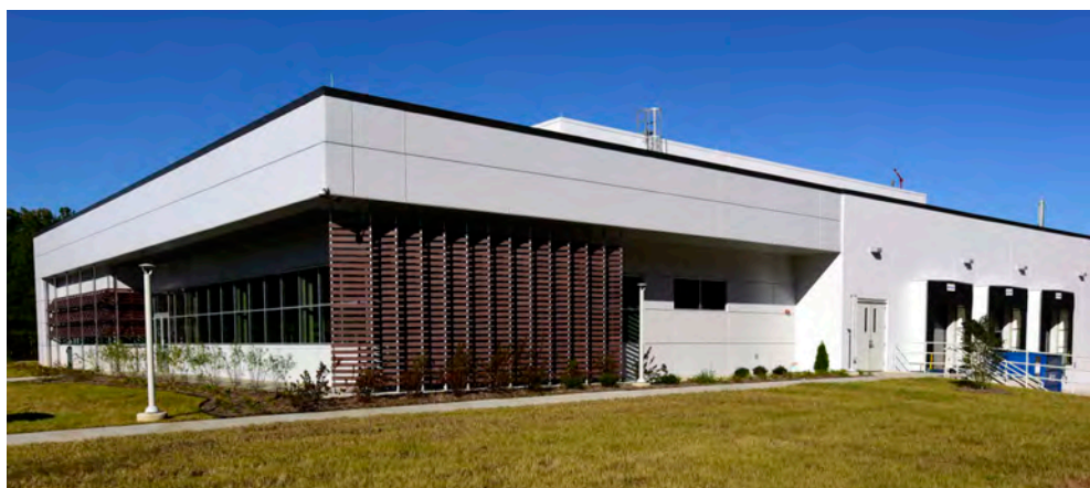
The warehouse features south-facing office space for solar heating. Louvers admit winter light and shade the hot summer sun.
