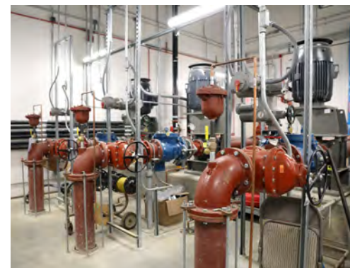
INSIDE THE PUMP HOUSES (from l): Water pumps in the TESS; the electrical vault supplying power to the TESS; and water pumps inside the IWSS. The pump houses outside both tanks are unoccupied and are operated remotely from the Central Utility Plant.
