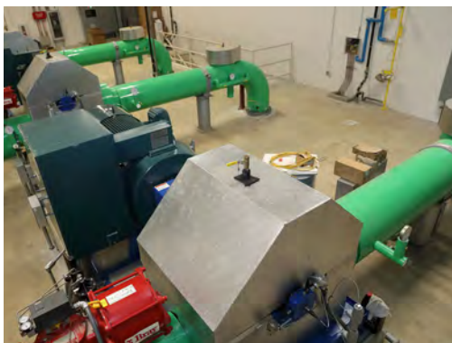
INSIDE THE PUMP HOUSES (from l): Water pumps in the TESS; the electrical vault supplying power to the TESS; and water pumps inside the IWSS. The pump houses outside both tanks are unoccupied and are operated remotely from the Central Utility Plant.
