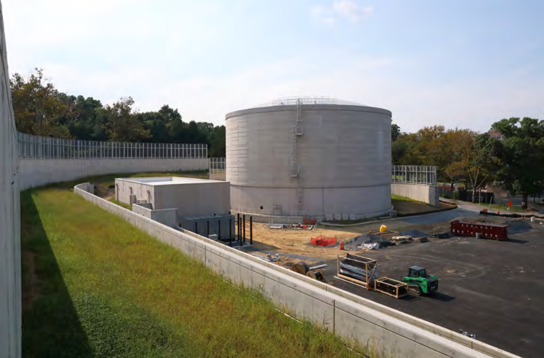
At left, the IWSS is flanked by a massive concrete retaining wall, with parking lot 42 adjacent to it. At right is the TESS exterior, featuring the temperature sensors. Data from these sensors are used to calculate the thermocline level in the tank—the contents' temperature at different heights within the cylinder.
