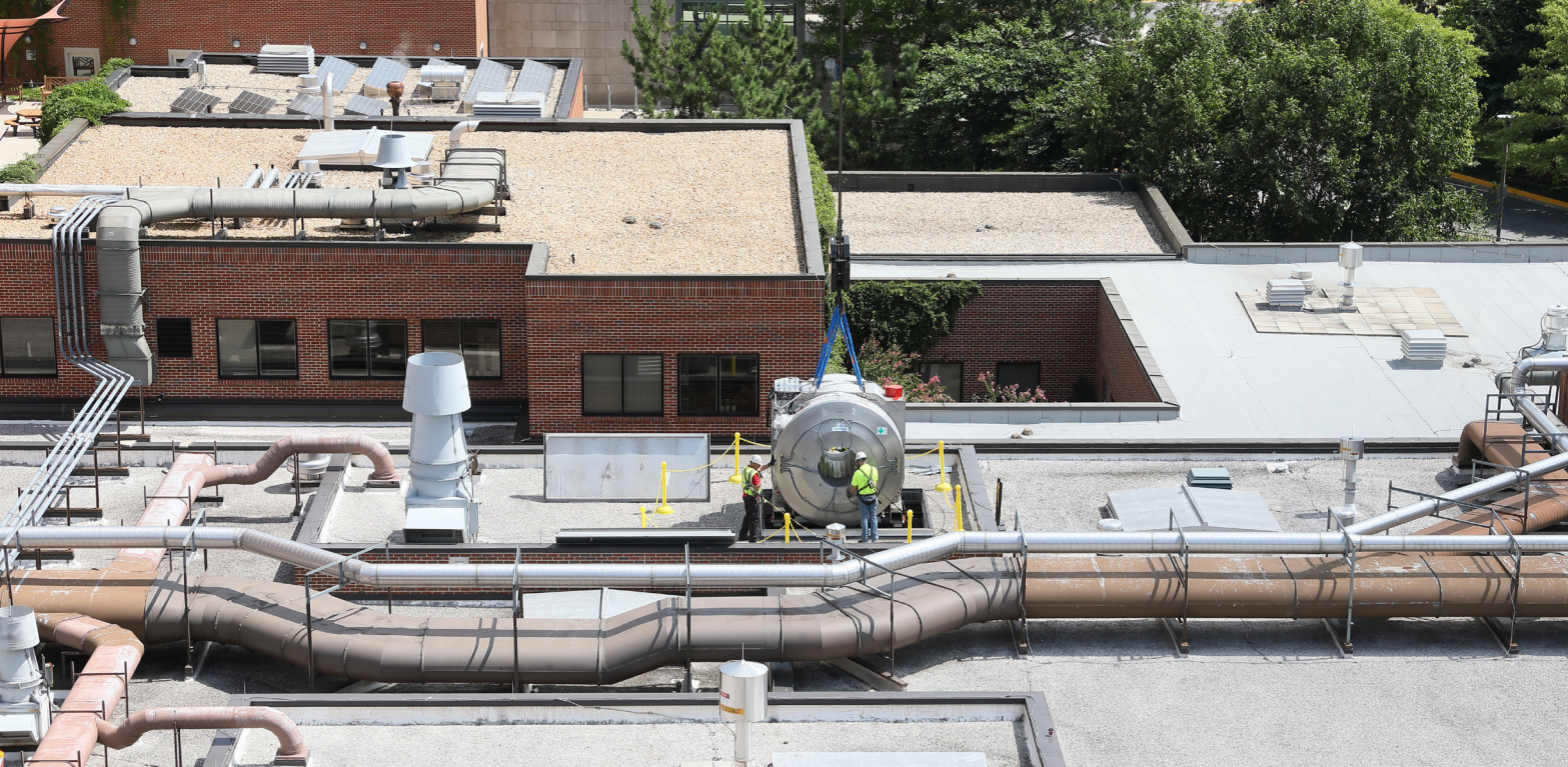
The 7T magnet eases through a roof hatch, with an inch to spare on each side. There are also bay doors in the side of the facility that can admit magnets.
