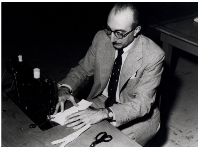
DeBakey stitches a Dacron graft artificial artery at home, on his wife's sewing machine in 1955. One of DeBakey's most important surgical innovations was the Dacron vascular graft, which he developed to replace sections of blood vessels damaged by aneurysms, especially in the aorta.
