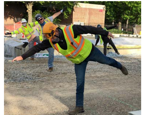
Not the Hokey Pokey. Construction Safety Week aims to keep workers healthy on the job site. See more on p. 12.
