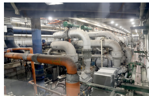
Above, CUP control room view of half of 60,000-ton chiller plant; below, Memarzadeh (r) points out CUP features.
