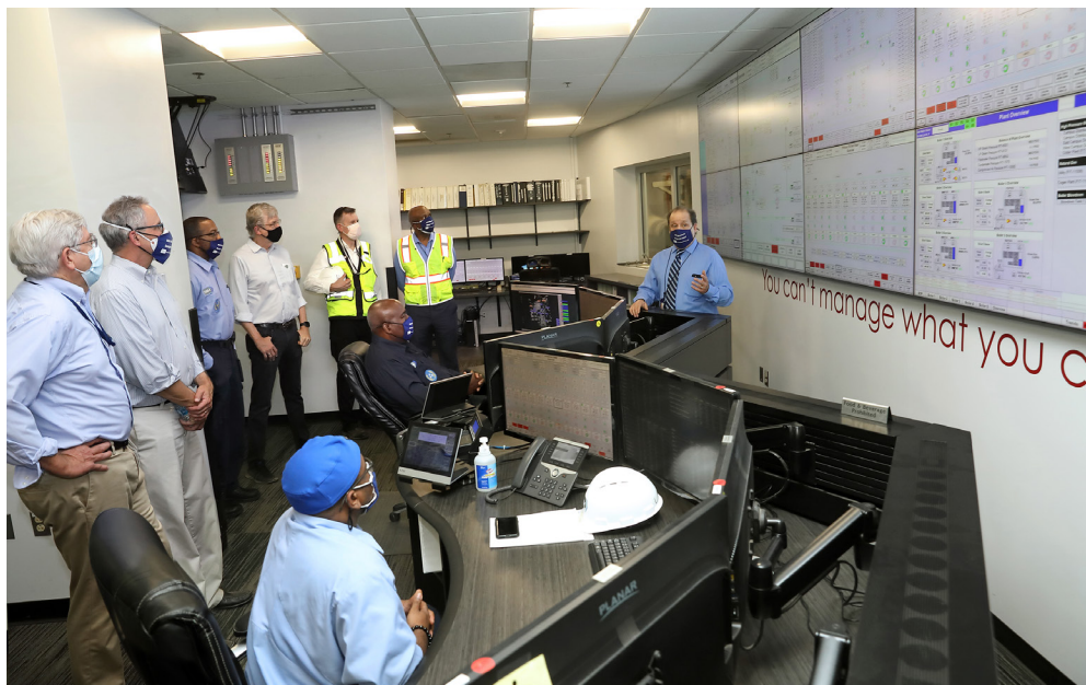
Wall of screens: CUP staff monitor operations in real time from the control room shown above.
