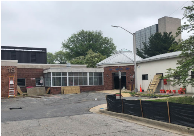
Bldg. 18 sits empty, awaiting demolition.
