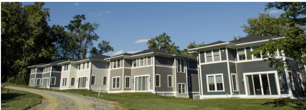
A view of the back of four new FAES houses along Cypress Avenue
