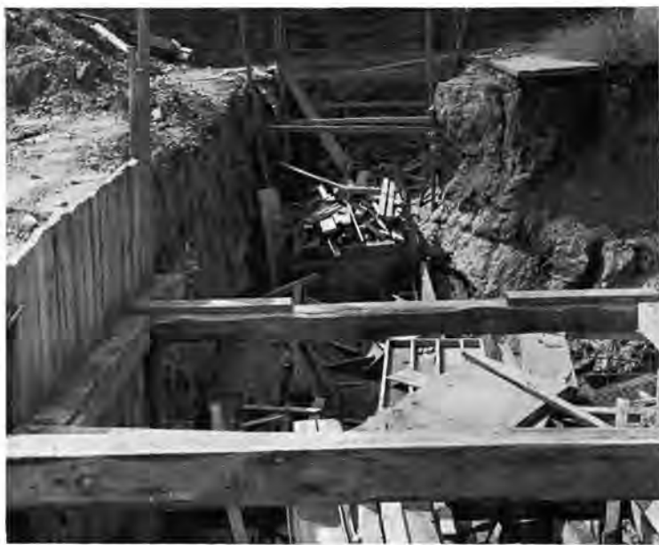
ON THE MORNING AFTER the flooding of the pipeline trench, the section extending to the north wall of the power plant (Bldg. 11) looked like this. It was through this portion of the wall that the water penetrated. Note the debris from dislocated shoring and the high-water mark, indicated by the top line of the lighter earth on the bank at right.
