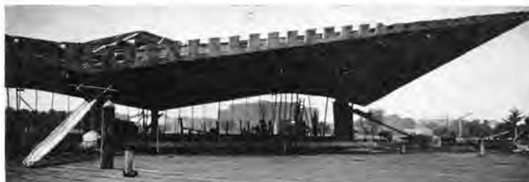
This recent picture, looking northwest, shows a portion of the hyperbolic paraboloid shell under construction atop the new National Library of Medicine Building here.—Photo by Bob Pumphrey.
