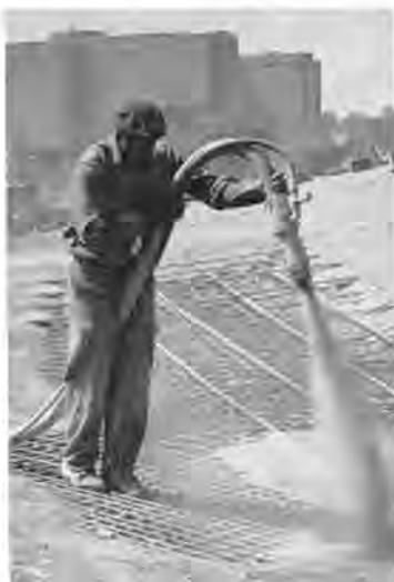
A workman on top of the hyperbolic paraboloid shell that crowns the National Library of Medicine Building sprays Gunit concrete onto the steel reinforcing between ribs of the shell.—Photo by Sam Silverman.
