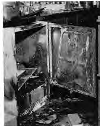
This refrigerator was totally destroyed and adjacent cabinets were partially damaged in an explosion and fire in Building 4.
