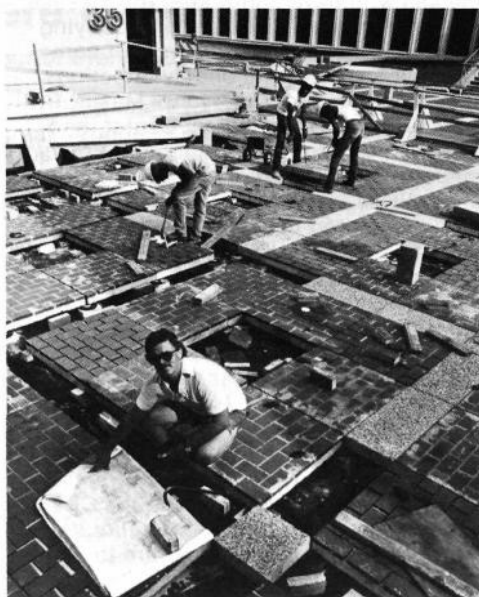
Foreman Ramon Hart of Universal Management checks blueprints for the laying of the terrace brick around Bldgs. 35, 36, and 37.
