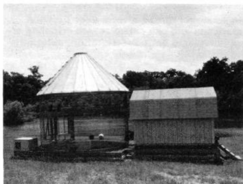
A particularly attractive feature of the new primate research facility is the outdoor preserve, where the monkeys are free to come and go as they please.
